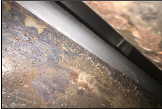
Before: Worn leading edge of wicket gate.
