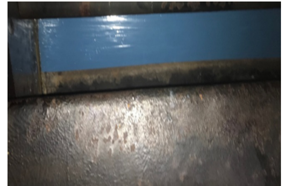
After: Final topcoat of ARC SD4i.
