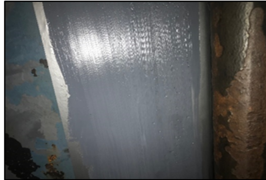
In process: Application of ARC 858 rebuild coat.
